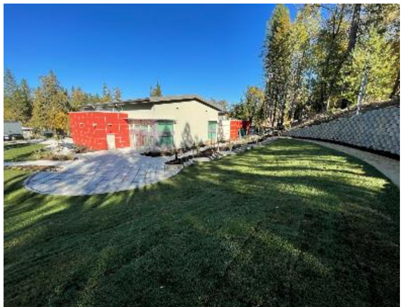
New sod and outdoor lighting are completed at the grass amphitheater for the Groveland Resilience Center
