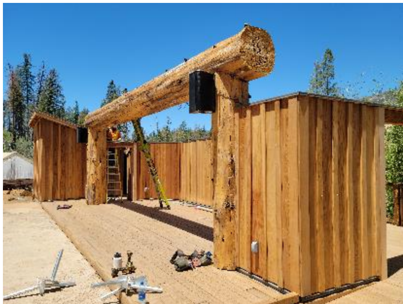
Work under way at the Tuolumne Berkeley Camp Amphitheater
